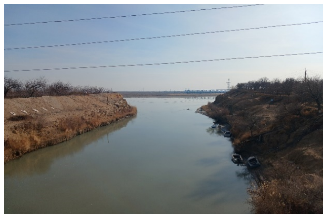
(c) The entrance to the Tashsaka intake structure itself.
