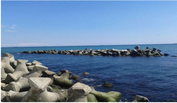
Figure 5. Detached Breakwaters – Longitudinal structures
